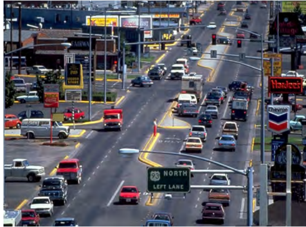
Incomplete streets can create a dangerous environment for people outside of cars.
